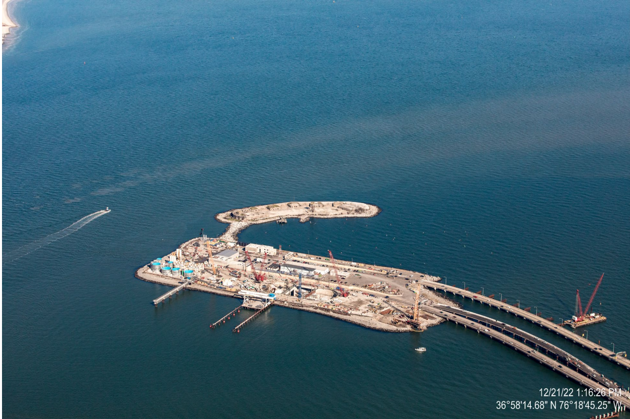
South Island Construction Activities Associated with the Expanded HRBT. Source: VDOT
